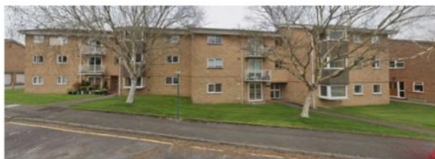
Fig. 1. Front street view of Block B, 26-54 Beverley Court. Adapted from Google Maps.
