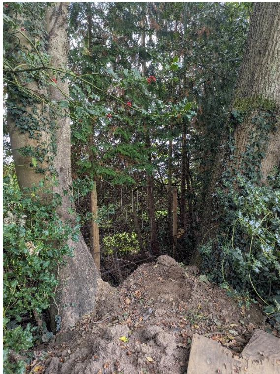
Photograph of the debris at the base of T52 and T53.
